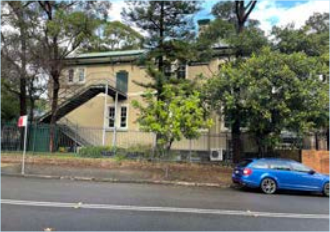
Kegworth Public School on Lords Road (South)
