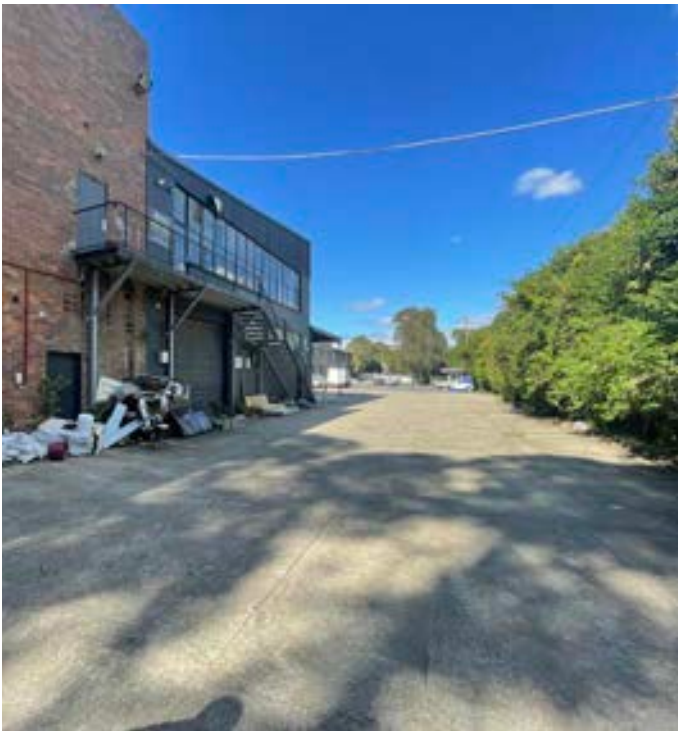
2. North-western corner looking south
